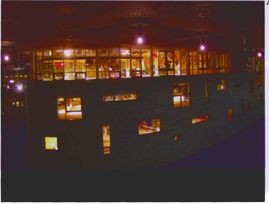
7 The facade of the Schiffsbau culture and media centre Medio Rhein.Erf. The parabol-shaped form of the Municipal Library is located between the City Hall and the extended culture and media centre of the city: which means an ideal location in the heart of Bergheim.
